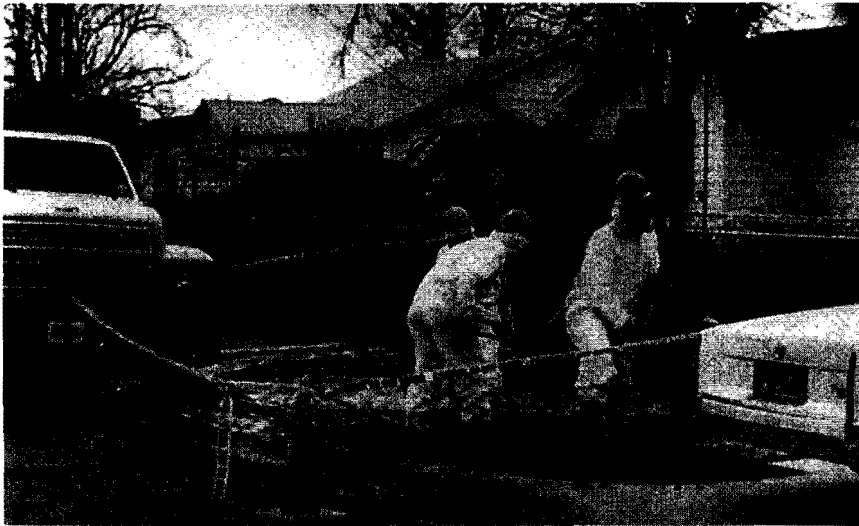
Crews begin cleanup of lead-tainted soil in West Dallas, Texas, neighborhood, 1992. (Photo by Luis D. Sepulveda, president of West Dallas Coalition for Environmental Justice)
