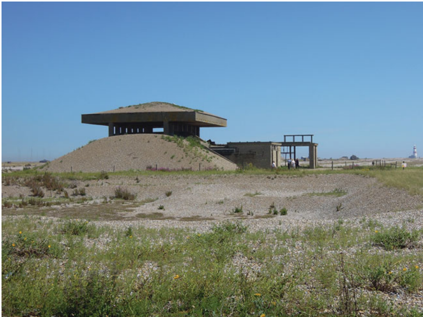
Fig. 9.3 Orford Ness and the 'Pagoda' Nuclear Weapons-Testing Facilities. (Photo: Simon Wellings, all-geo.org . Reproduced with permission)
