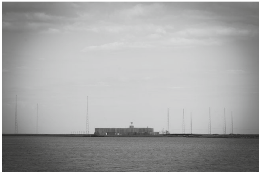
Fig. 9.2 The Orford Ness secret ‘Cobra Mist’ project—designed to detect missile launches and aircraft movements in the Soviet Union during the Cold War. The aerials shown are part of an array originally covering 135 acres. The ‘blockhouse’ building on the bank of the River Ore was the project’s control centre. The general public is still denied access to the site. Source: Andrew Houston
