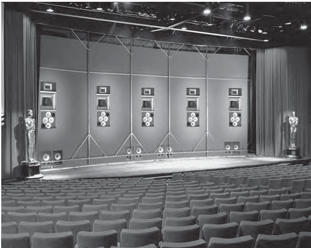
FIGURE 16.2 The Samuel Goldwyn Theater in the Academy of Motion Picture Arts and Sciences, Hollywood, California, with the screen down and showing the five front channels and subwoofers, all JBL loudspeakers. Photo courtesy of JBL Professional; “Academy Award” and “Oscar” image © AMPAS®. THX® Lucasfilm, LTD.
