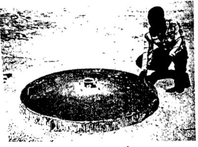
Making of the cover slab of a pump. The concrete is poured in the mould half full, then the reinforced bars are placed on top. Later the mould is filled with concrete. The bolts have to reach the reinforcement bars in order
