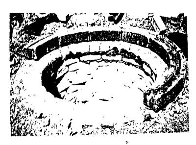
The outside diameter of this well is 1.2 m. Since the diameter of our cover slab is 1.5 m, the diameter of the well has also to be increased to that of the cover slab. In doing this normal bricks were placed differently as can be seen then, inter locking blocks were used to enlarge the diameter.
