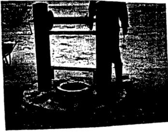
Making of the cover slab and the windlass. It is done in two parts 1. the cover slab and the man hole. 2. windlass stand.
