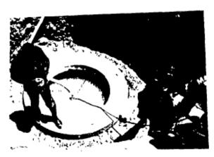
The foundation of this well is made of collar placed on a hard rock.
