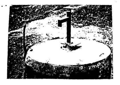
Installation of the pump. The pipes are connected out side the well and placed inn. This is how it look like after the connection is done.
