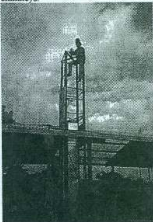
Construction of the Nicaraguan chimney
