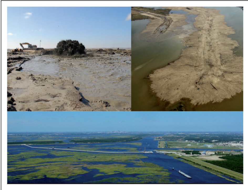
Figure 3. Top: The “beneficial use” of material dredged from the Mississippi River includes building landforms near the river’s mouth to mitigate coastal land loss. Below: A storm surge barrier built in 2011 across the intersection of two shipping canals near New Orleans (skyline in distance). These canals, legacy projects that date to the era of the Panama Canal’s opening in the early 20th century, have been contested since Hurricane Katrina. The deeper canal was decommissioned and closed off in response to political pressure. Photos courtesy of US Army Corps of Engineers, New Orleans District.
