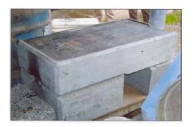
This cement Justa is being built by Helps International in the Guatemalan Highlands. Three individual cement pieces are cast in fiberglass molds and then assembled on site. The molds are easy to transport and prevent design inconsistencies.
