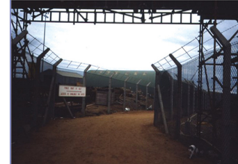
Sizewell Beach during the construction of Sizewell B
